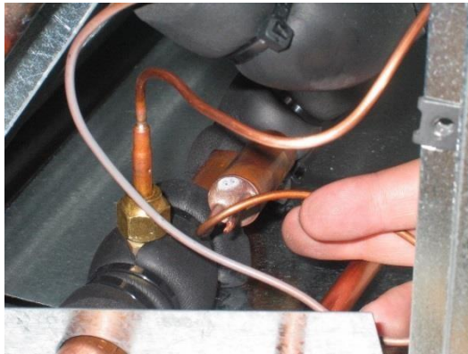
Figure 28. Thermal Measuring Bulb Placed on Copper Tube.
