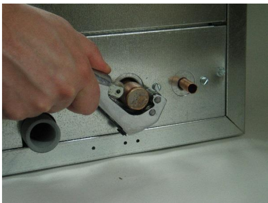
Figure 21. Cut end of connection as shown.
