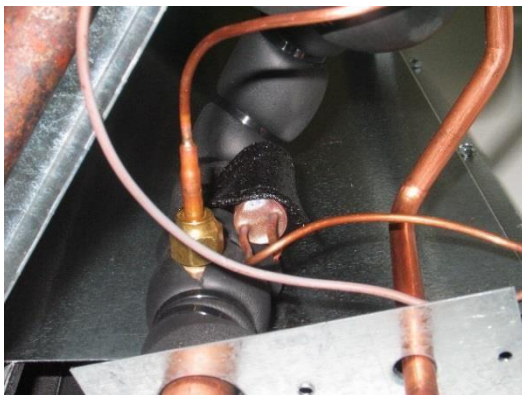
Figure 29. Bulb Secure Clamp and Cork Tape
