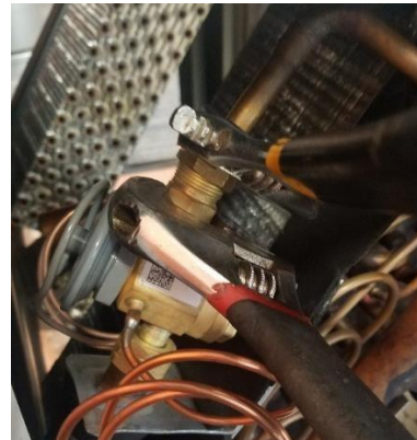
Figure 25. Attach and tighten upper connecting nut (B/E coils)
