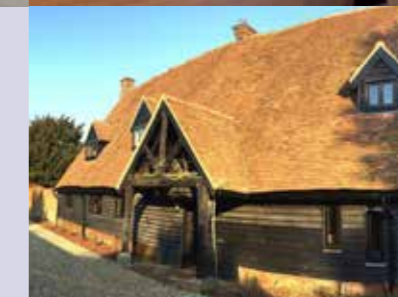
Retro fit to a historic property
