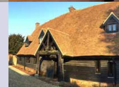
Retro fit to a historic property
