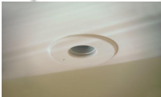
To provide both air conditioning and heating using a heat pump as the source, the Unico System features a heat pump coil. Air is pulled across the coils to provide either cool or warm air. Each apartment has its own system, whilst some of the larger apartments have two.
